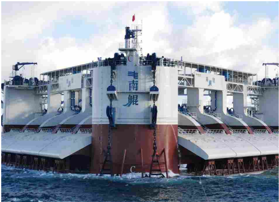
我国首兆瓦级漂浮式波浪能发电装置锚泊定位系统 China's first megawatt-scale floating wave energy power generation device uses a mooring positioning system
